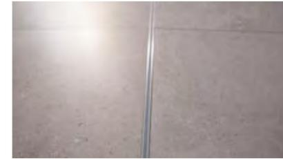
11- Take account of structural joints. Movement joints should be positioned as directed by the project designer. In general, do not design areas greater than 50-70 m2 for interiors and half that for exteriors. Minimum joint width: 8 mm.
