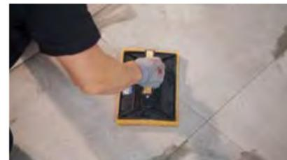
16- Wait for the grout to start to dry, then clean with a sponge dampened in clean water. Do not allow the grout to harden on the tile, especially on textured tiles. Do not soak the joint with excess water.
