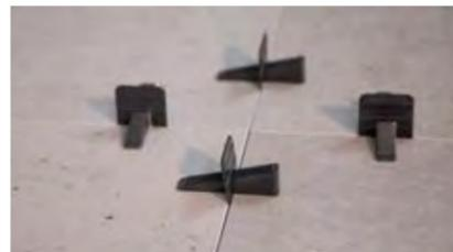
8- Grout joints should be at least 1mm for interior flooring and 5mm for exterior paving. For installations with offset joints, stagger the tiles at the 3/4 point. Self-levelling tile spacers are recommended.
