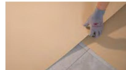
17- Protect the paving against premature loading, other construction work and adverse weather. We recommend covering the paving with sheets or boards to avoid a build-up of dirt and to protect from scratches, abrasion and impact.
