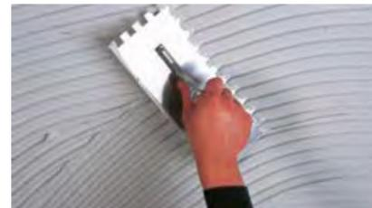
6- The only fixing system recommended is installation on a thin layer using a toothed trowel. A double bonding technique (with adhesive applied to both the substrate and the back of the ceramic tile) is recommended for tiles with a format larger than 1,000 cm2 (33x33 cm).
