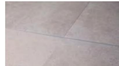
14- Joints should be grouted when the tiles are completely fixed to the substrate. In respect of paving, follow the recommendations of the adhesive manufacturer to ensure sufficient time is allowed before the floor is walked on or subjected to load. In this way movement and/or breakages are avoided.
