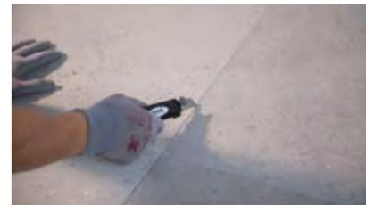
13- Prior to grouting, check that the bonding material has hardened. Remove the tile spacers, clean the joints along their length, width and depth, and check the joint is not damp.
